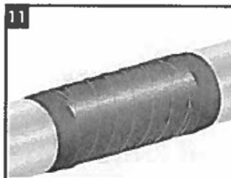
Allow the Wrapid Shield XL to reach a Shore D Hardness of 70 prior to pulling. Wrapid Shield XL is fully cured at a Shore D Hardness of 83 @ 72°F.
