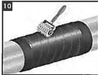
Perforate the compression film using a wire brush (or other perforating device) by lapping firmly on the tape with the metal bristles. Perforation allows the CO<sub>2</sub> gas generated by the curing process to escape. Compression film may be removed after material hardens and either discarded or left in place.
