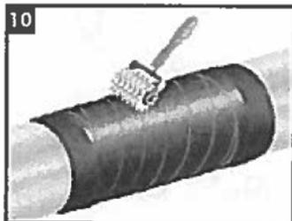
Perforate the compression film using a wire brush (or other perforating device) by tapping firmly on the tape with the metal bristles. Perforation allows the CO<sub>2</sub> gas generated by the curing process to escape. Compression film may be removed after material hardens and either discarded or left in place.
