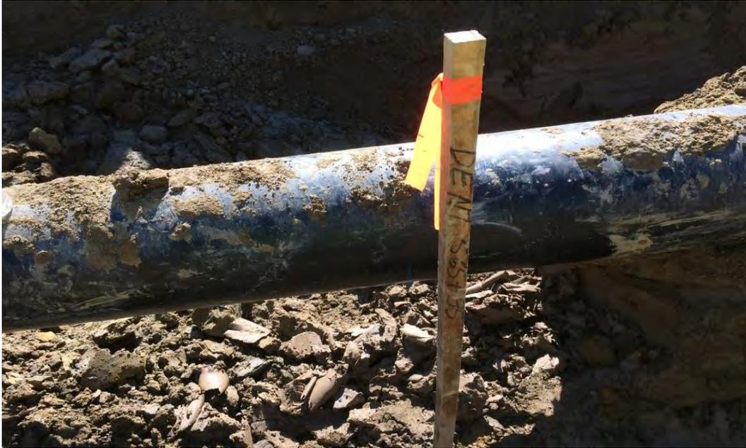
No dent or coating damage spotted at station 565+85 after cleaning the pipe and thoroughly inspecting the pipe by hand. Checked the pipe several feet upstream and downstream of station number.
