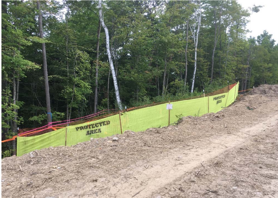
Photograph 1: Harsh sunflower area within Project corridor marked by high visibility green fencing with "Protected Area" lettering.
