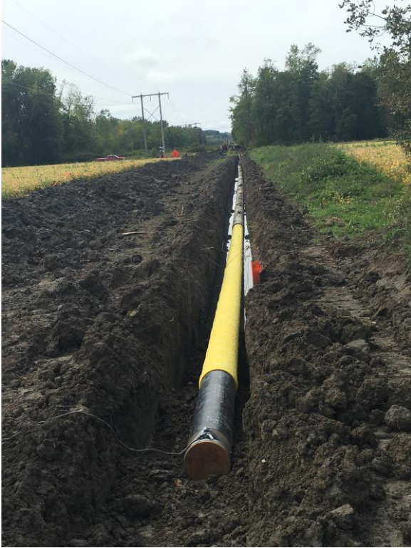
Photograph 5: Pipe installation leading into the Red Maple/Green Ash Swamp.
