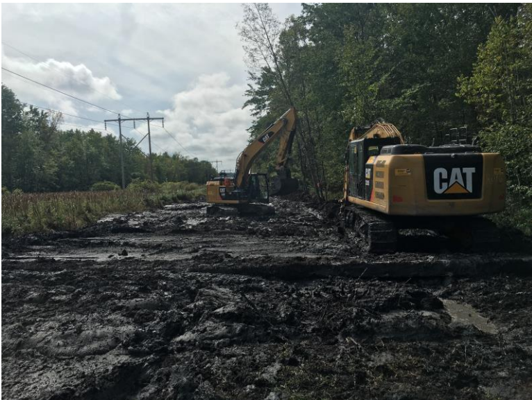
Photograph 6: Conditions were extremely challenging in the Red Maple/Green Ash Swamp. Crews continued to work off timber mats and managed to keep materials within the work limits to the best of their ability.
