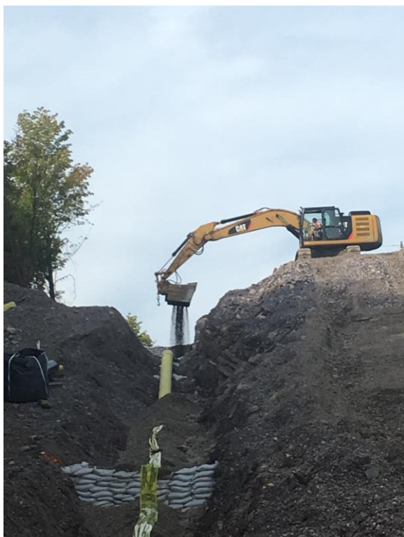
Photograph 2: Backfill between Hollow Road and Post Road in Monkton. Trench breaker shown in foreground. Utilizing shaker bucket to sift out material being placed in the backfill.
