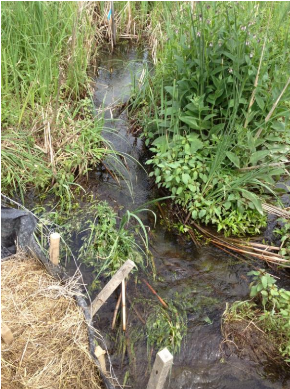
Photograph 4: High flows in wetland behind silt fence adjacent to the area shown in Photograph 3 above. Water was visibly clear and no turbid discharges were observed leaving the construction site.
