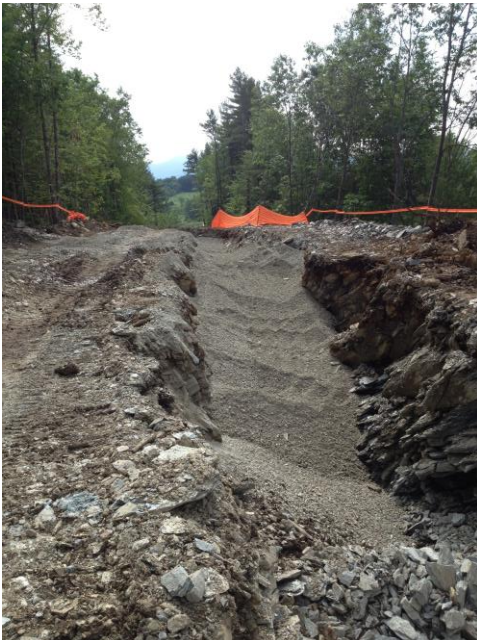
Photograph 2: Trench backfilled with processed (crushed) 1 ½" minus material.
