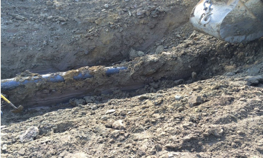
Exposing more pipe to weld 0193. No rocks detected just clumps of clay and clay topsoil mix.
