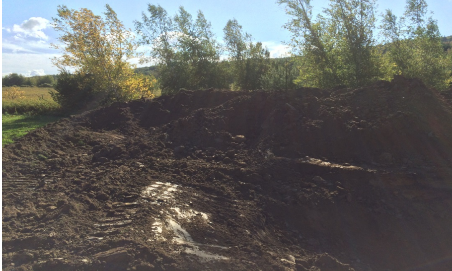
Excavation dirt pile with clumps of clay and no rocks.
