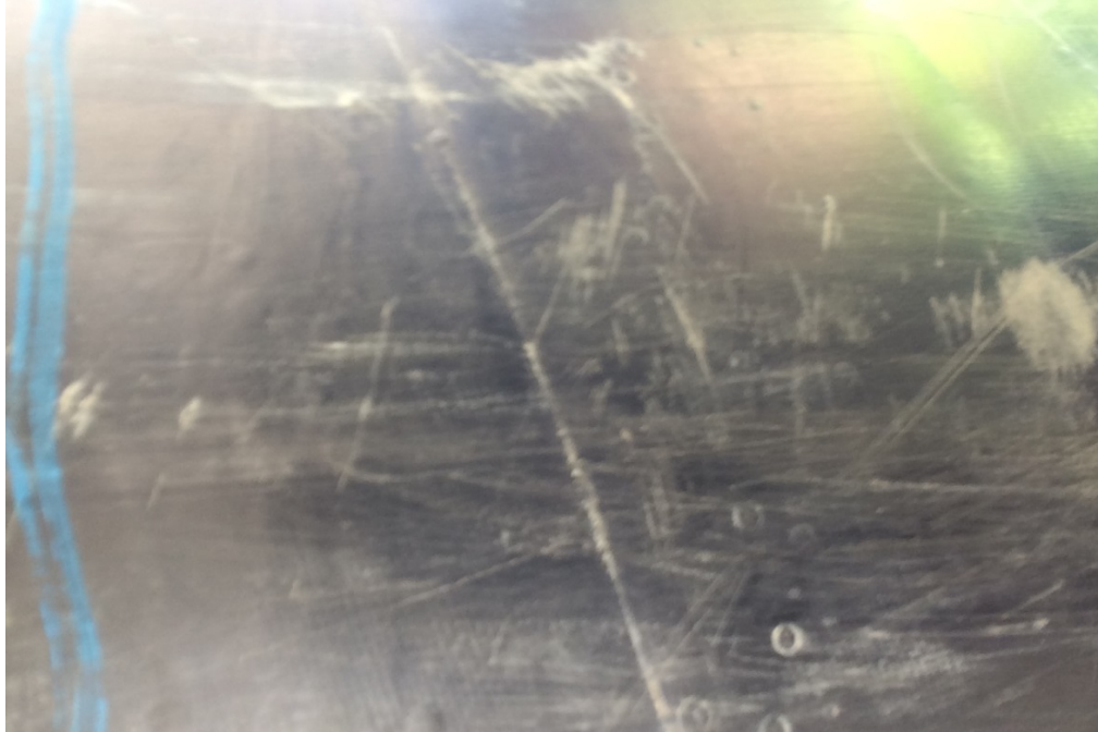
Close up picture of station 565+85 at the 4:00/4:30 location. No coating damage or dent detected
