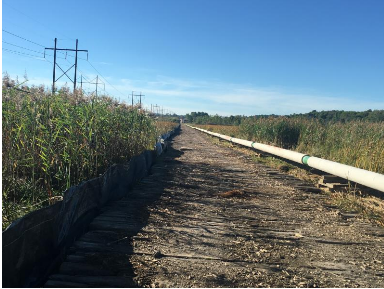
Photograph 7: New Haven Swamp viewed from the north facing south. No excavation to date.
