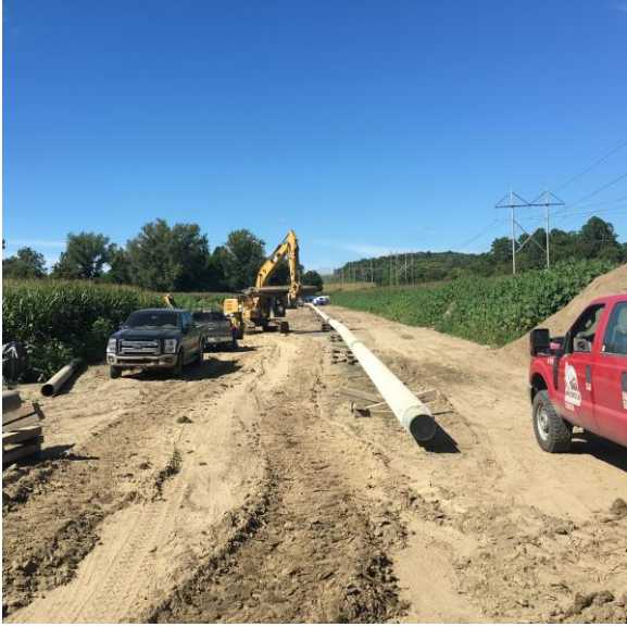
Photograph 9: River Road tie-in to the New Haven River HDD.
