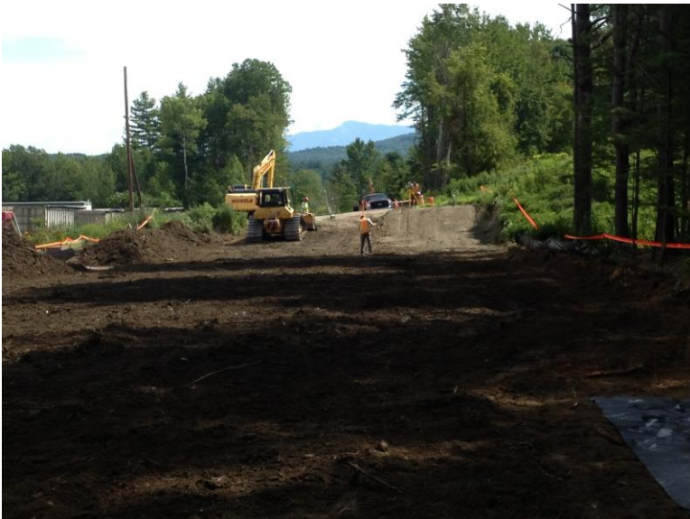
Photograph 2: Michels Pipeline Construction stripping topsoil between stations 393+00 to 396+00.
